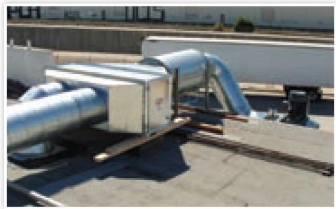
Exhaust duct from the DustHog SFC downward flow dust collector with in-line silencer and safety filter.
