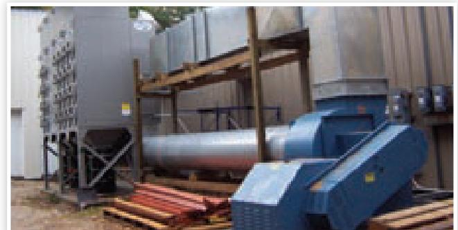
A SFC 48-4 with an air distribution module and ground mount blower collects plastic dust.
