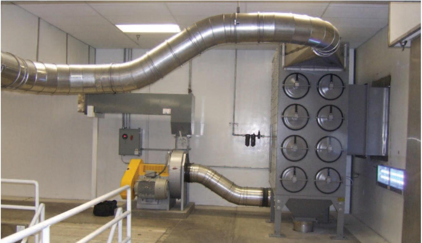
**Dust collectors with explosion venting can safely be used indoors with venting through an exterior wall, as shown here.**
