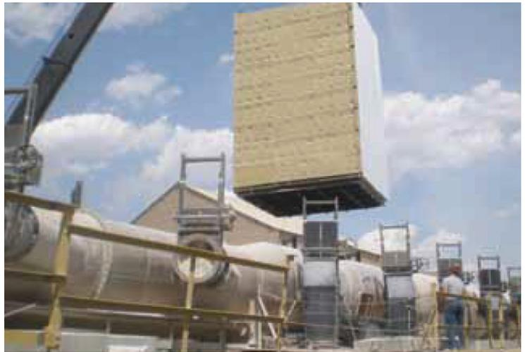
**Figure 2:** difficult crane access required 'flying' half of the compartments over the on-line system. Careful planning and close co-ordination were required to assure the compartment change-outs went smoothly
