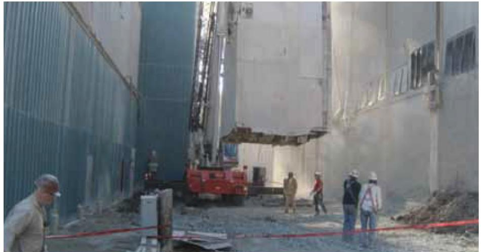
Figure 1: the tight access made the removal of individual compartments difficult.
